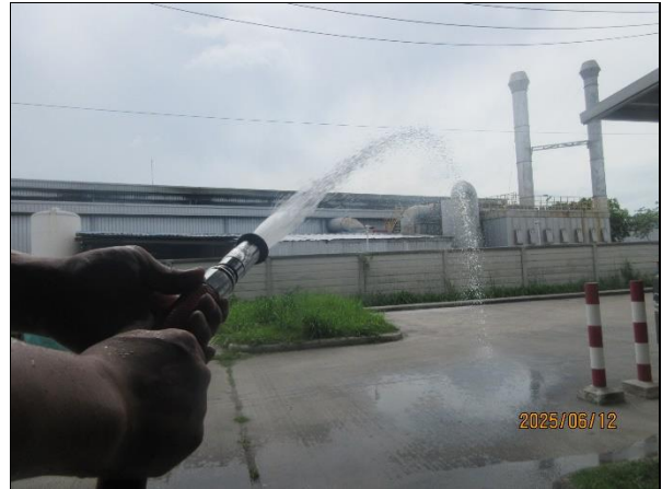
Fire hydrant testing
